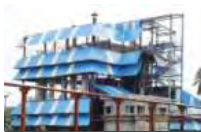
900m 3 / Day 5 Effect Falling Film Evaporator and Spray Dryer – IFB Agro Industries Ltd. (West Bengal), INDIA
