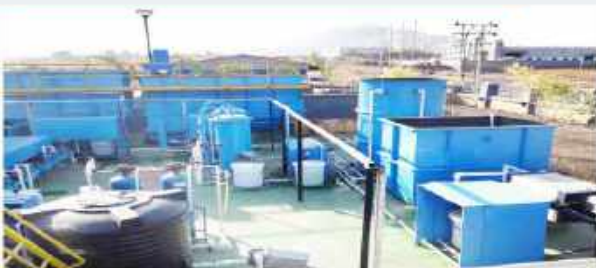
Condensate Polishing Unit (CPU)
