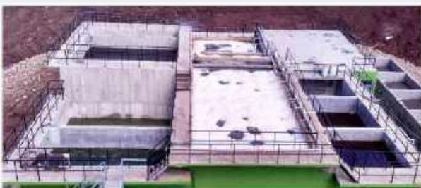
Condensate Polishing Unit (CPU)
