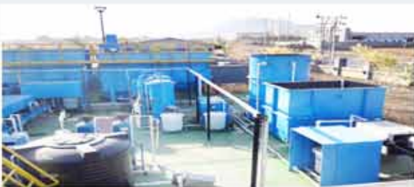
Condensate Polishing Unit (CPU)
