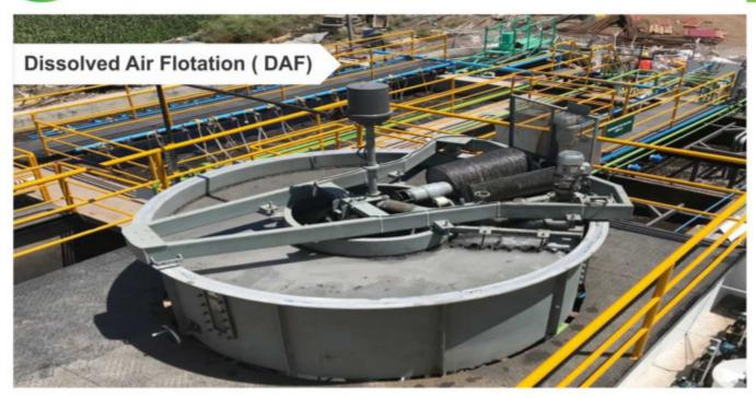
In The DAF unit suspended solid, Fat, Emulsified & Free Oils are removed from effluent. Here chemical are dosed from dosing tanks. Air Compressor and HPP are provided for this system.
