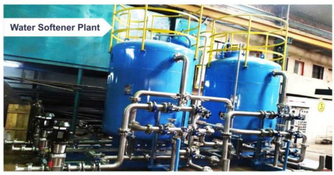
Water softening is the reduction of the concentration of Calcium, Magnesium, and other ions in hard water. We offer highly durable Water Softening Plant that is used to exchange ions through resin bed in Sodium form and providing suitable soft water. The resin bed is regenerated using common salt solution for regaining its ability after a certain period.
