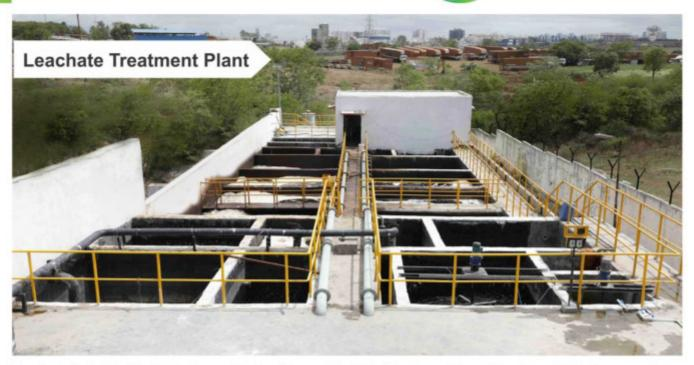
Leachate is the liquid that drains or 'leaches' from a landfill of garbage Depot. It varies widely in composition regarding the age of the landfill and the type of waste that the garbage contains. It usually contains both dissolved and suspended material which pollutes the environment.
