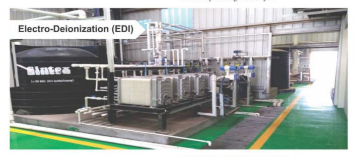
Electrodialysis is a process in which electrically charged membranes are used to separate ions from aqueous solutions under the driving force of an electrical potential difference. Because of the arrangement of ion-selective membranes, the migrating ions become concentrated in each alternate cell in the stack.
